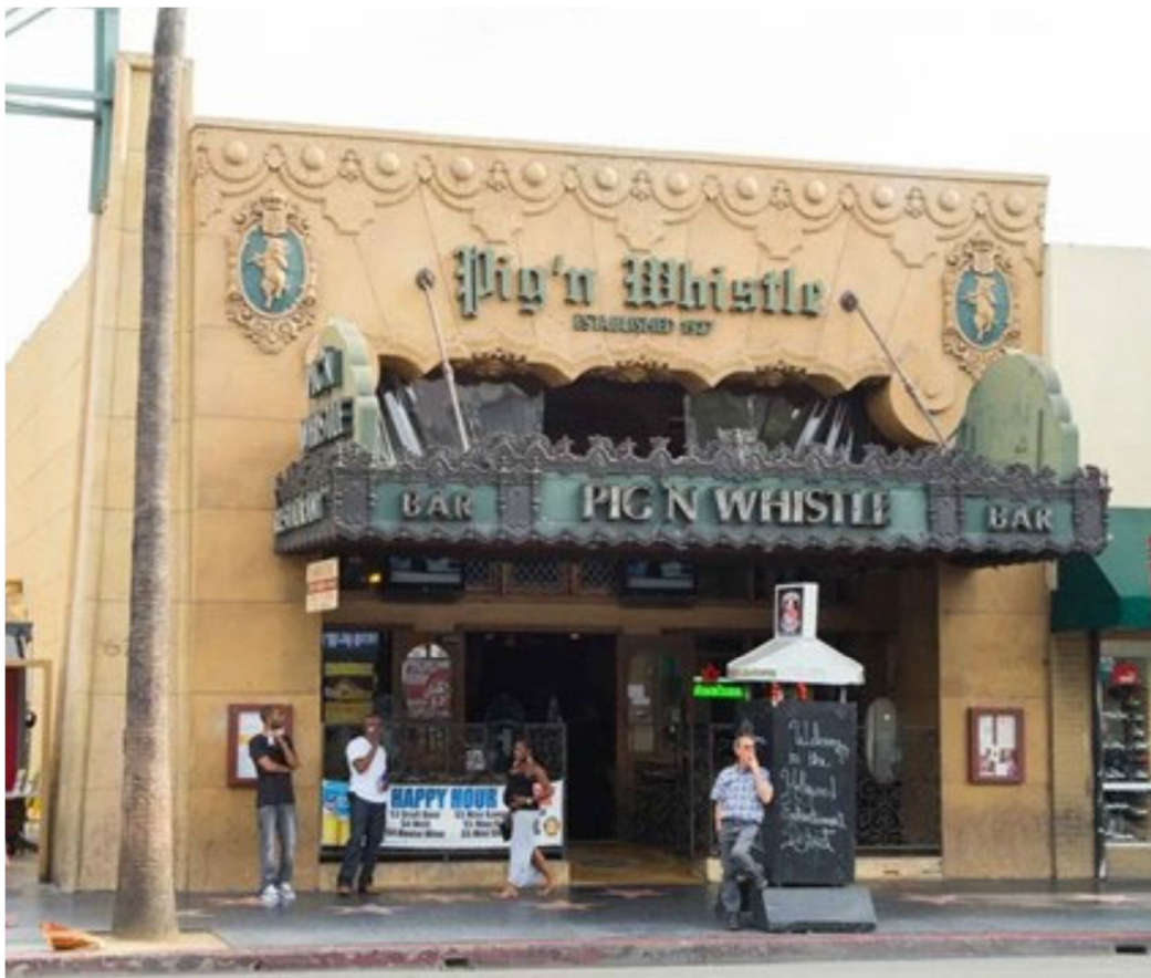
Figure 6 - MFR Report Figure 9 dated 2014. “The marquee was restored as part of the 1999–2001 renovation, including reconstruction of the side fins with neon-lit channel signage. The extant channeled neon signage was added at that time. SOURCE: Photo provided by Sunset Entertainment Group.
